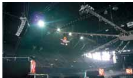
Zurich's Hallenstadion with the PA of DYNACORD V-System enclosures as well as DYNACORD H5000 and Electro-Voice TG7-amps
